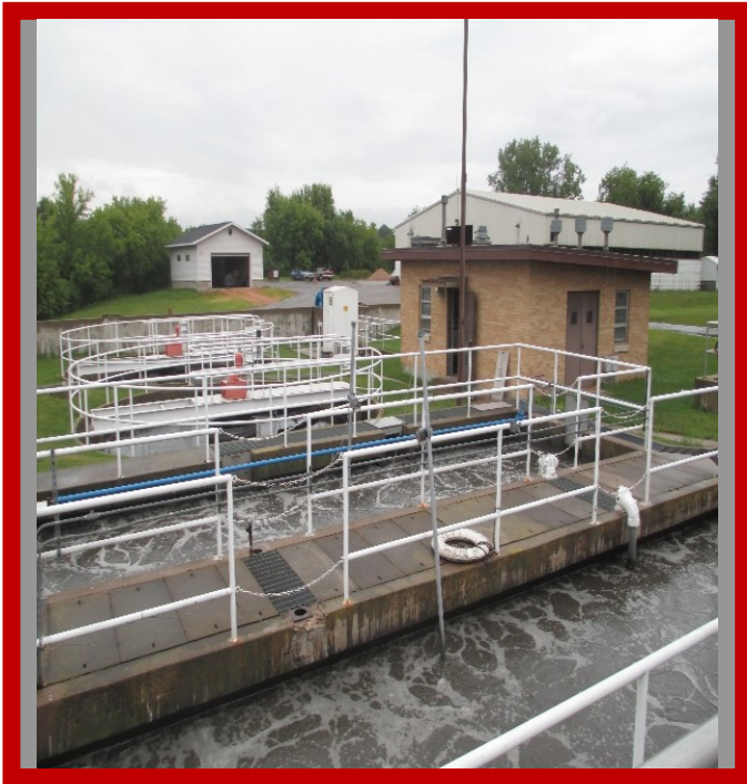
Existing Wastewater Treatment Plant
